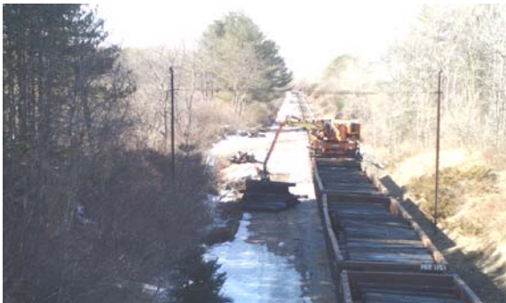
Pan Am crews have started distributing ties for spring installation.
