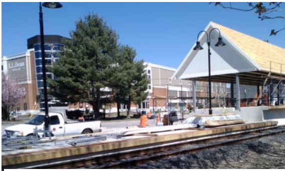
Freeport platform construction is progressing.
