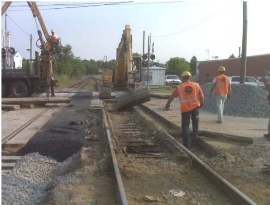
Congress Street Grade Crossing Reconstruction July 19, 2011
