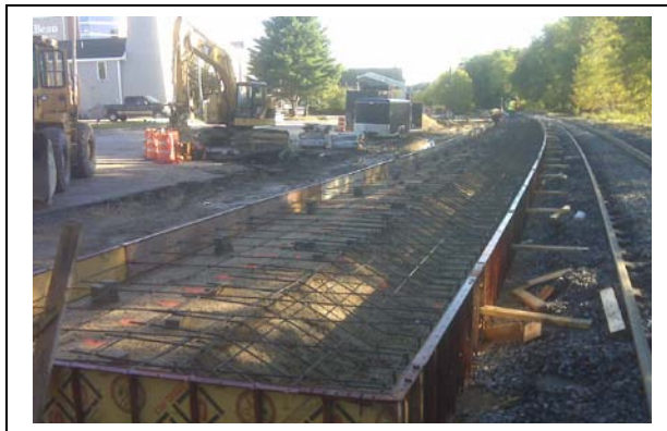
Construction of the Freeport Platform began September 1, 2011
