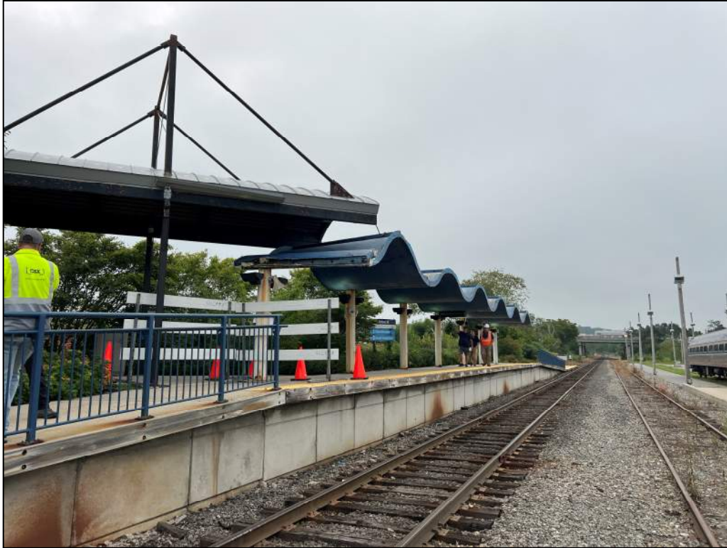
Photo 3 – Existing Canopy and Platform Configuration
