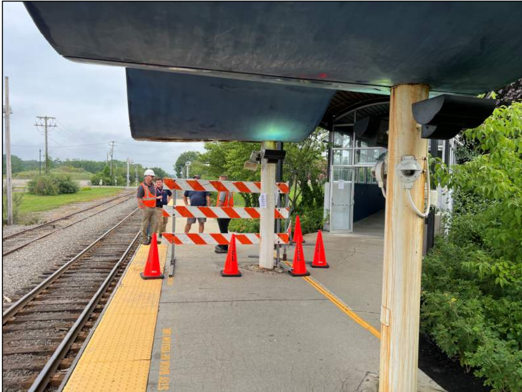
Photo 1 – Existing Canopy and Support Column Adjacent to Trainway
